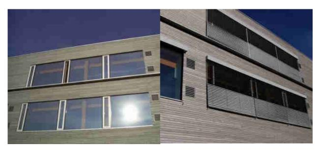
Figure 25 Missing external shading in the first year (left picture) caused overheating in the classrooms of the New Secondary School Schwanenstadt. As reaction to this an external shading system was installed in the second year (right picture).
