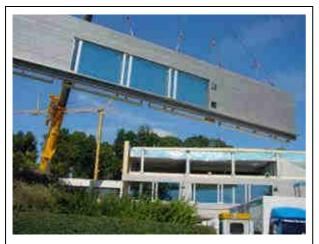
Figure 1 Integrated wooden frame windows and solar shading in a big prefabricated timber module for renovation of a school façade (Source: PAUAT Architekten)
