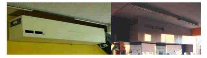
Figure 26 Missing housing of decentralised ventilation units caused sound problems in the first operated model classroom (see left picture). The housing was installed regularly later (right picture) to improve the situation in the classrooms.
